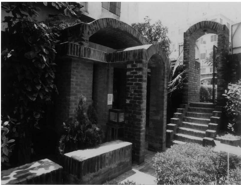
The stairs to enter the site are also an entry down memory lane. Courtesy of the Liberation War Museum.
