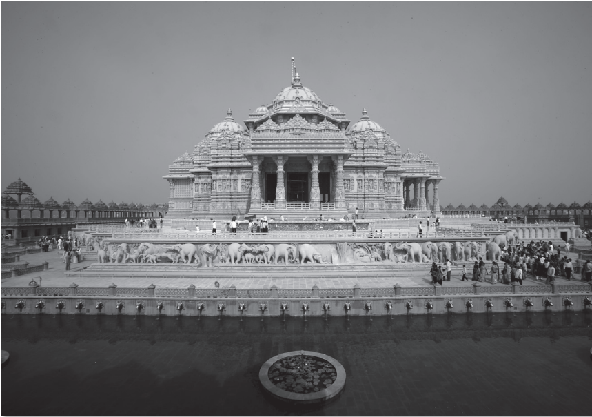
Akshardham, a Hindu temple-cum cultural complex, recently built in New Delhi. Courtesy of BAPS,* New Delhi/Ahmedabad..
