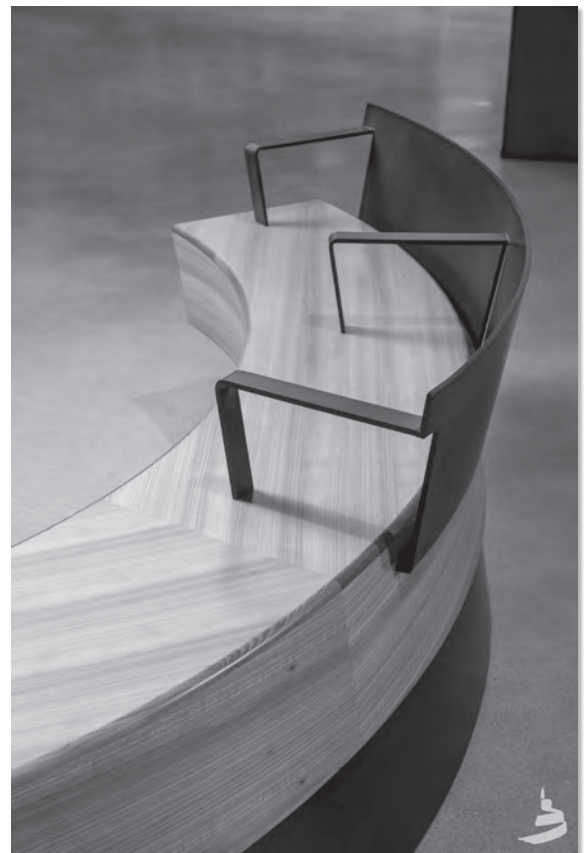
Fig. 2. The benches provide back support and arms for increased accessibility—the ability to push up and out of a seat—and fit the aesthetic and design approach. Courtesy of the Canadian Museum for Human Rights
