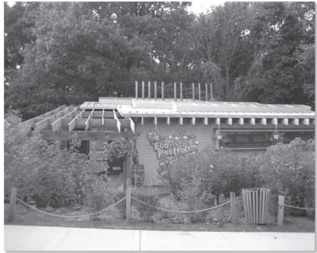
The Eco-restroom project, located at one of the Bronx Zoo’s Park entrances, includes eco-friendly bathrooms, a grey-water garden, rainwater garden, and an extensive interpretation program. Photo courtesy of WCS.
