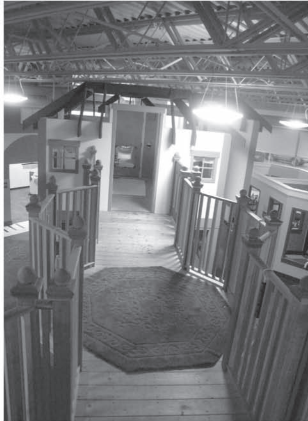
The “bell” on the bridge path allows two visitors using wheelchairs the chance to pass each other as they roll from either end of the bridge. It also provides groups of children with a place to pass each other. Courtesy of the Center for Creative Play.
