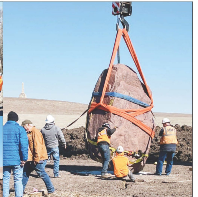
A HEAVY JOB - What was scheduled to be a one hour job Wednesday afternoon was more involved. Positioning the 28-ton Kaw Nation sacred prayer rock had its challenges, with four hours needed to place the rock. The rock was positioned on a 30-inch deep concrete pad, facing the The Kanza Monument, a 35-foot limestone tower that was erected by Council Grove citizens in 1925 as a tribute to the Kanza. The site is still considered to be a construction site and not ready for visiting as additional concrete work is scheduled for today.
