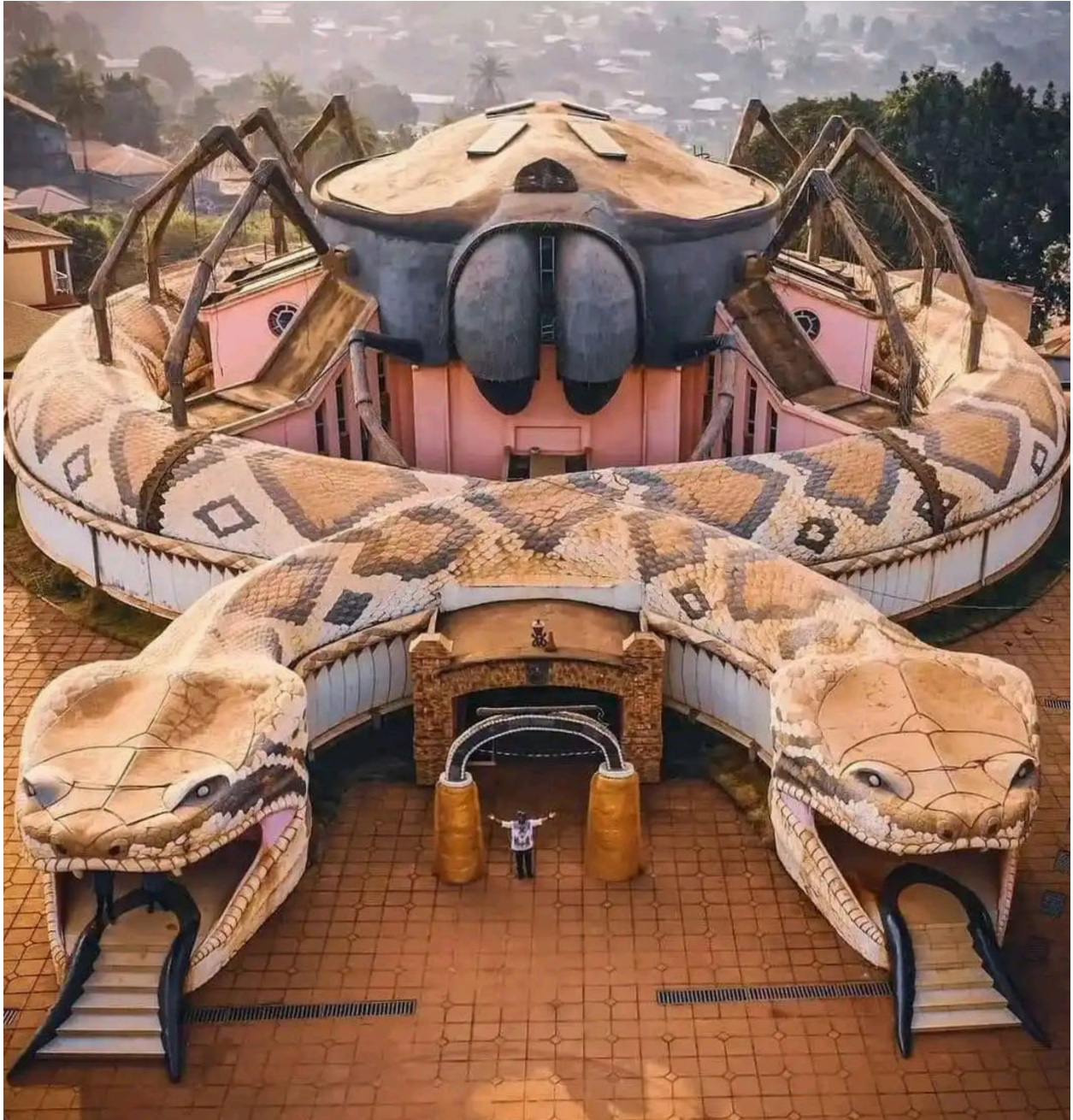
Figure 6: Exterior aerial view of the Bamoun Heritage Preservation Space la Musee des Rois in Fomban, Cameroon, designed on the community's cultural sensitivities and knowledge systems.
